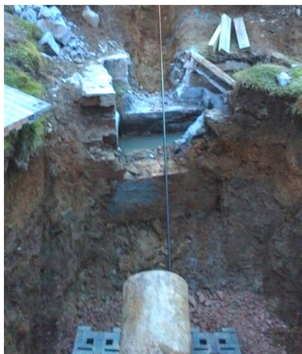
Figure 20. End pit with connection to gravity sewer
