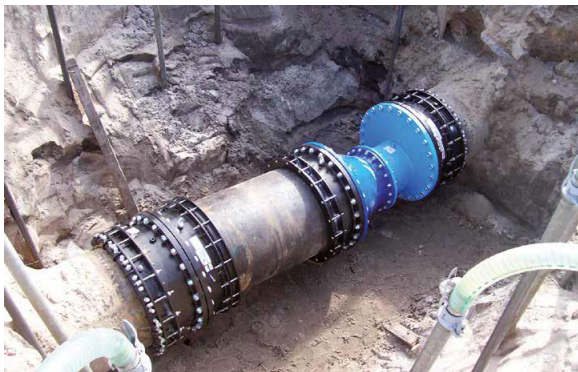
Figure 16 and 17. Reintegration of the Primus Line system® using spool pieces
