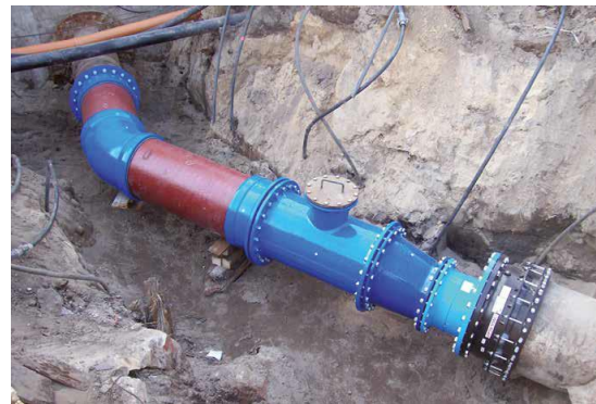
Figure 16 and 17. Reintegration of the Primus Line system® using spool pieces
